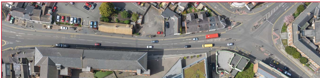
Aerial photograph of Lower Bond Street, Hinckley
