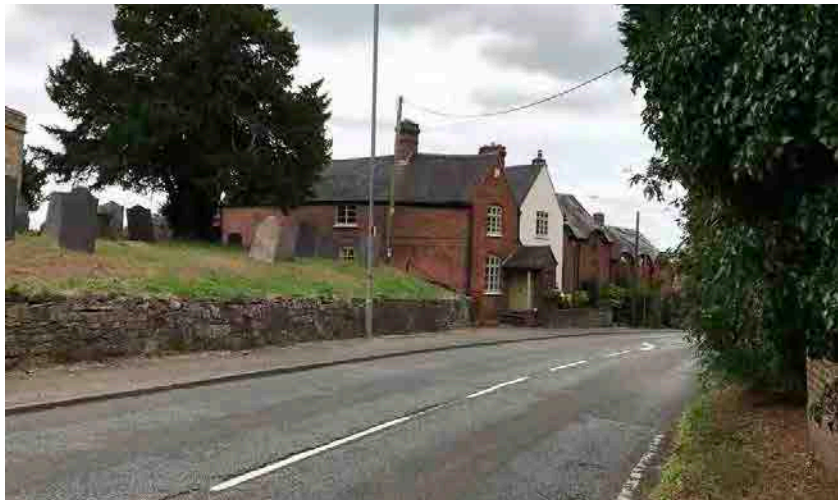
Properties in the setting of the church, Church Street
