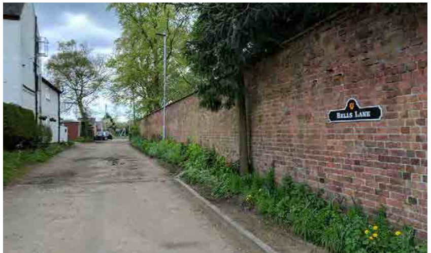
High brick boundary wall of the Rectory
