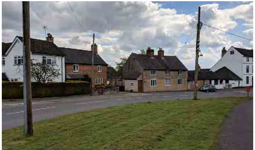
Main Street, incorporating characteristic smaller-scale cottages and farmhouses
