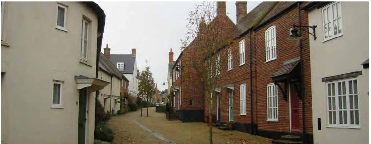
High quality design can be achieved in many ways. Above: The use of historic materials and architectural forms create the character of a traditional village at Poundbury, Dorset. Below: Contemporary design of buildings and landscape at Derwenthorpe, York, executed in high quality materials
