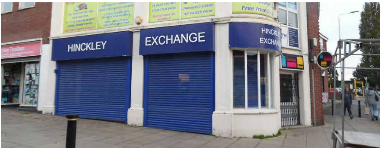
Above: Poor quality roller shutters: external shutters create inactive frontages outside of business hours. Below: Internal perforated shutters allow visibility, light and interest
