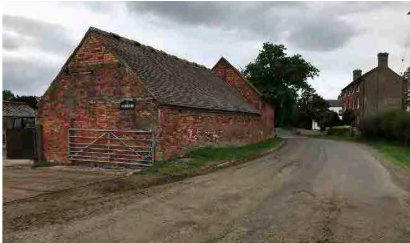
Manor Farm on Carlton Road, marking the southern approach to the village
