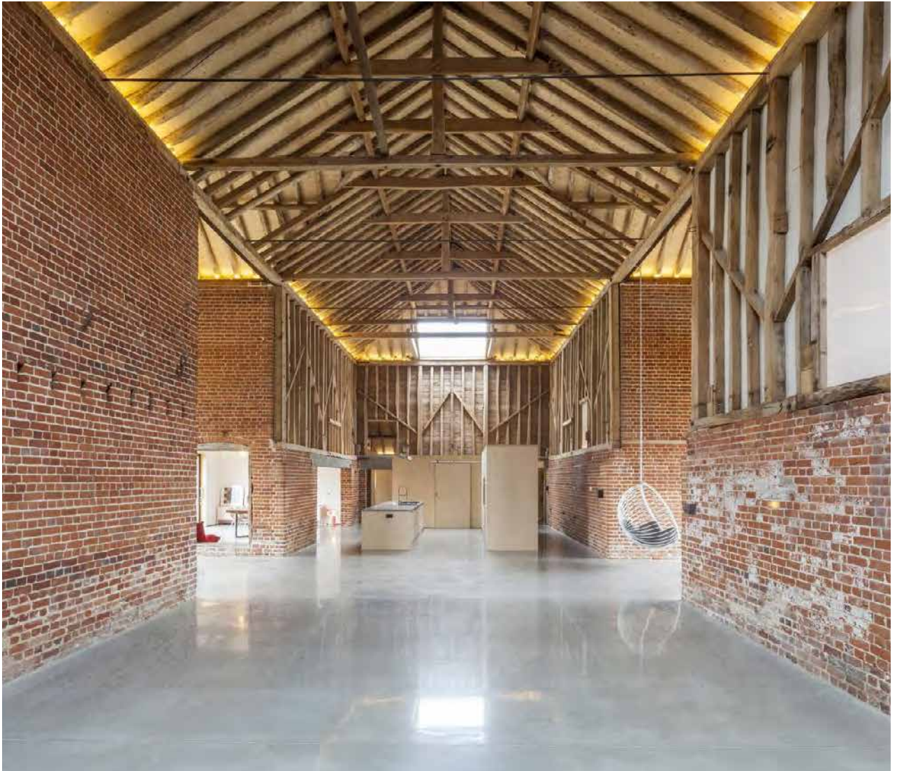
Above: In the interest of preserving character, conversions should avoid domestication of barn buildings. Below: Reuse of historic apertures can ensure continuity of character, with window frames set back within aperture where they are introduced
