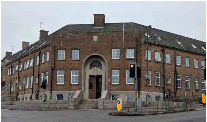
Early 20th century former police station, Upper Bond Street
