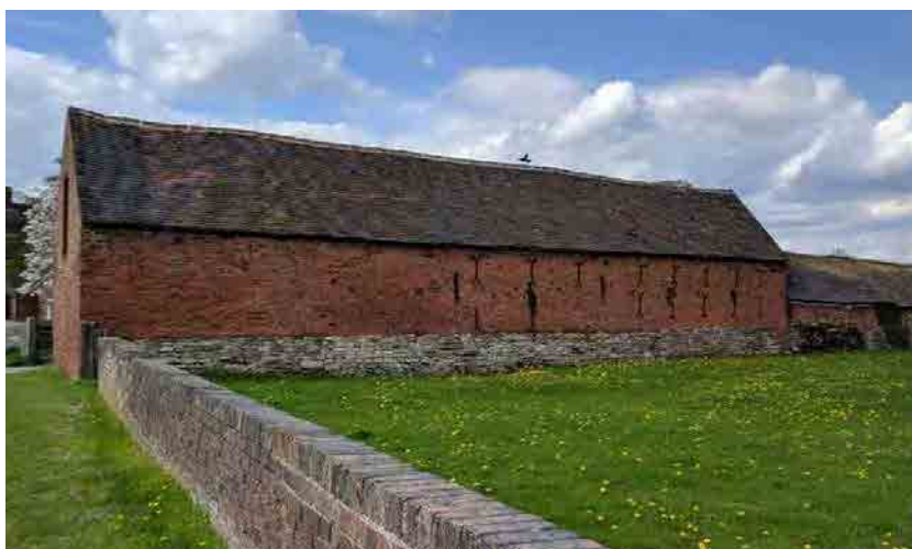
Farm building at the hamlet's centre along Main Street
