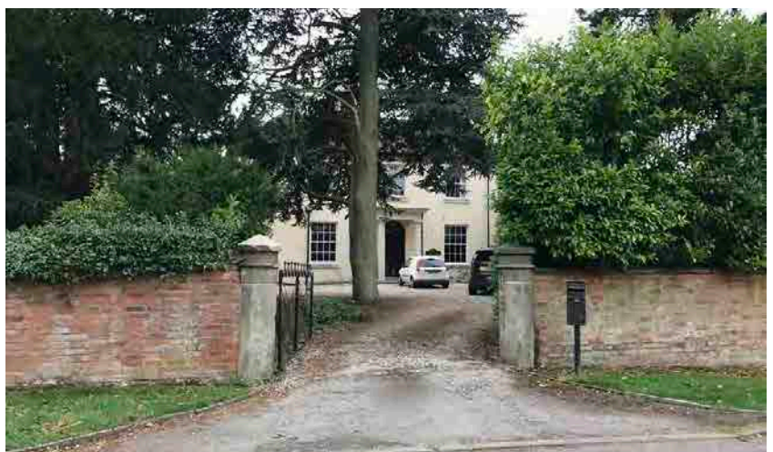
19th century former Rectory along Church Lane
