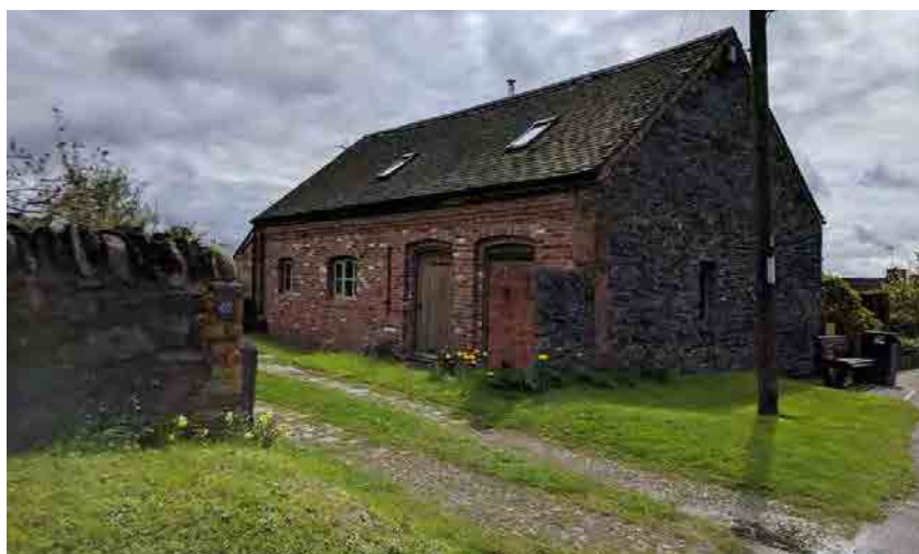
Farm buildings on Church Lane
