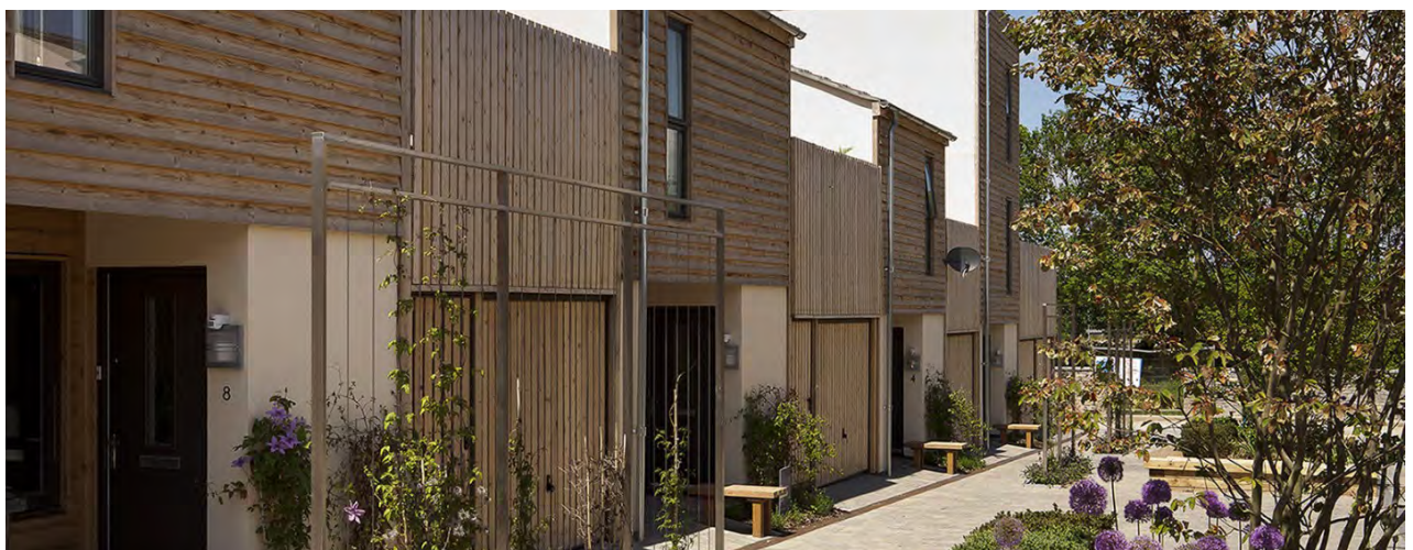
Figure 34 | The BfL award winning Lime Tree Square, Street, Somerset
