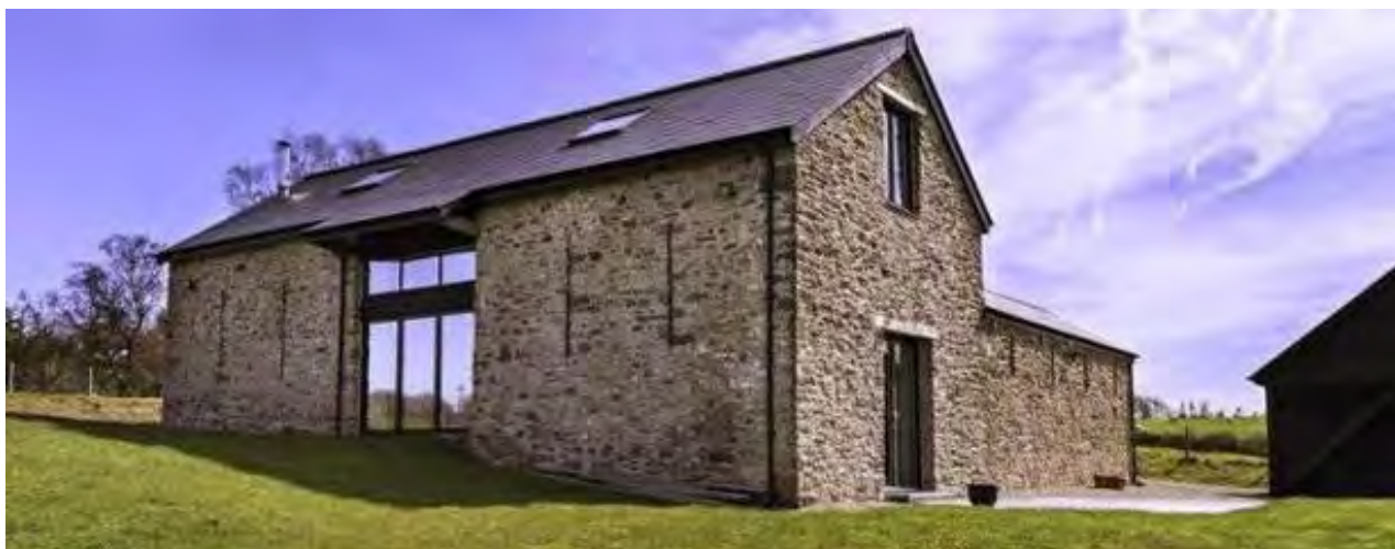
Above: External elevations avoid complexity, opting instead for decorative restraint. Below: retention of original doors and external features includes ventilation slots and metal ties. No new openings have been created and new windows and doors are of untreated oak. Re-roofing has worked with variations in the ridge to maintain character.
