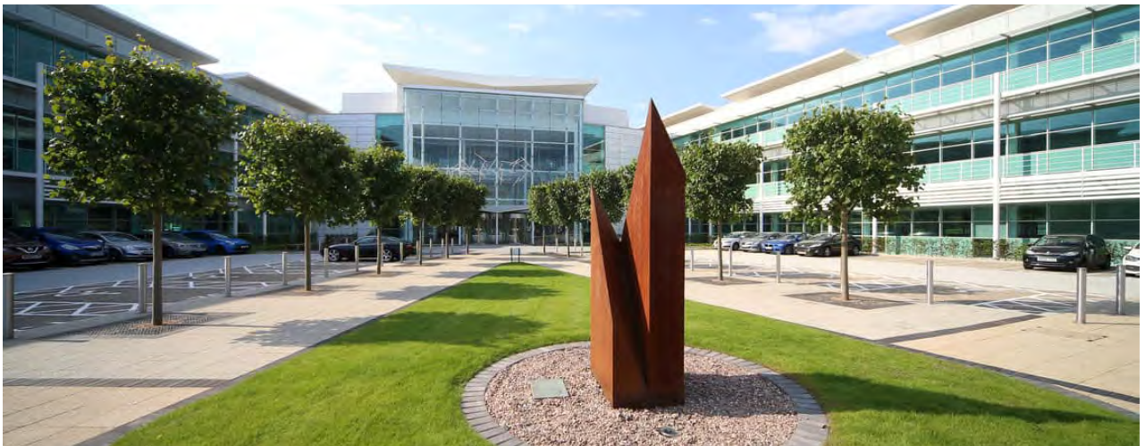
Use of quality materials and attention to detail in landscape design creates an inviting and attractive external environment at Blythe Valley Park in Solihull (photo: IM Properties). Below: Jaguar Land Rover, Wolverhampton. High-quality materials create a crisp and clean appearance
