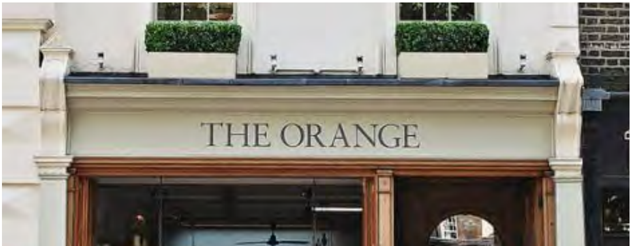
Above: Signage created through letters individually painted onto the fascia board. Below: Halo-illumination integrated to the underside of the cornice
