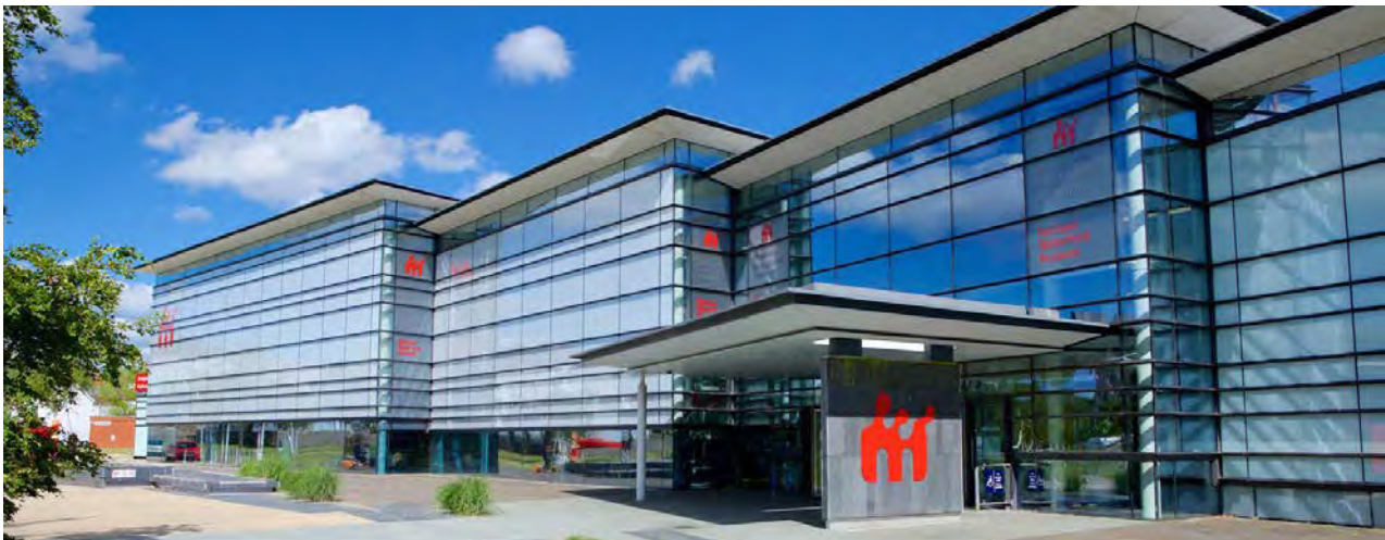
Above: The National Waterfront Museum in Swansea relates to its waterside location through its deliberately reflective choice of materials and wave-like forms. Below: Modern commercial development designed to reflect neighbouring historic factories through form and materials, Denmark
