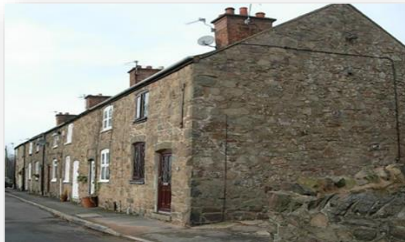
FIGURE 11: NEW ROW, HILLSIDE
