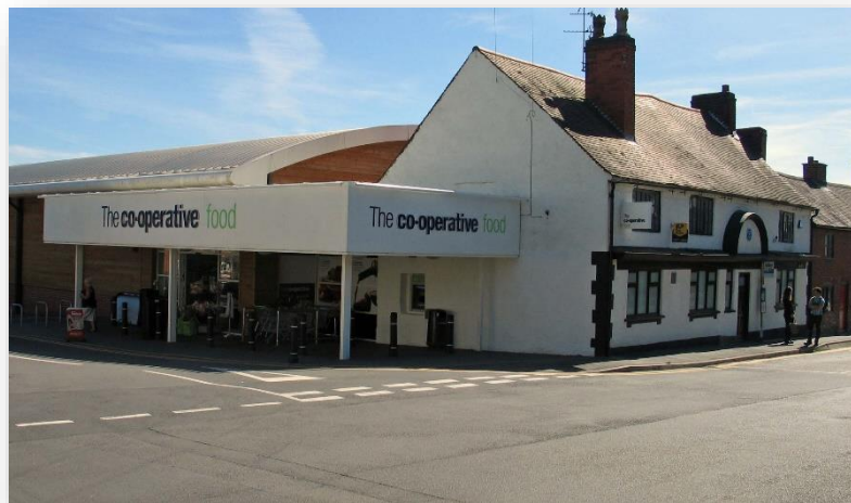
FIGURE 14: MARKFIELD CO-OP, MAIN STREET
