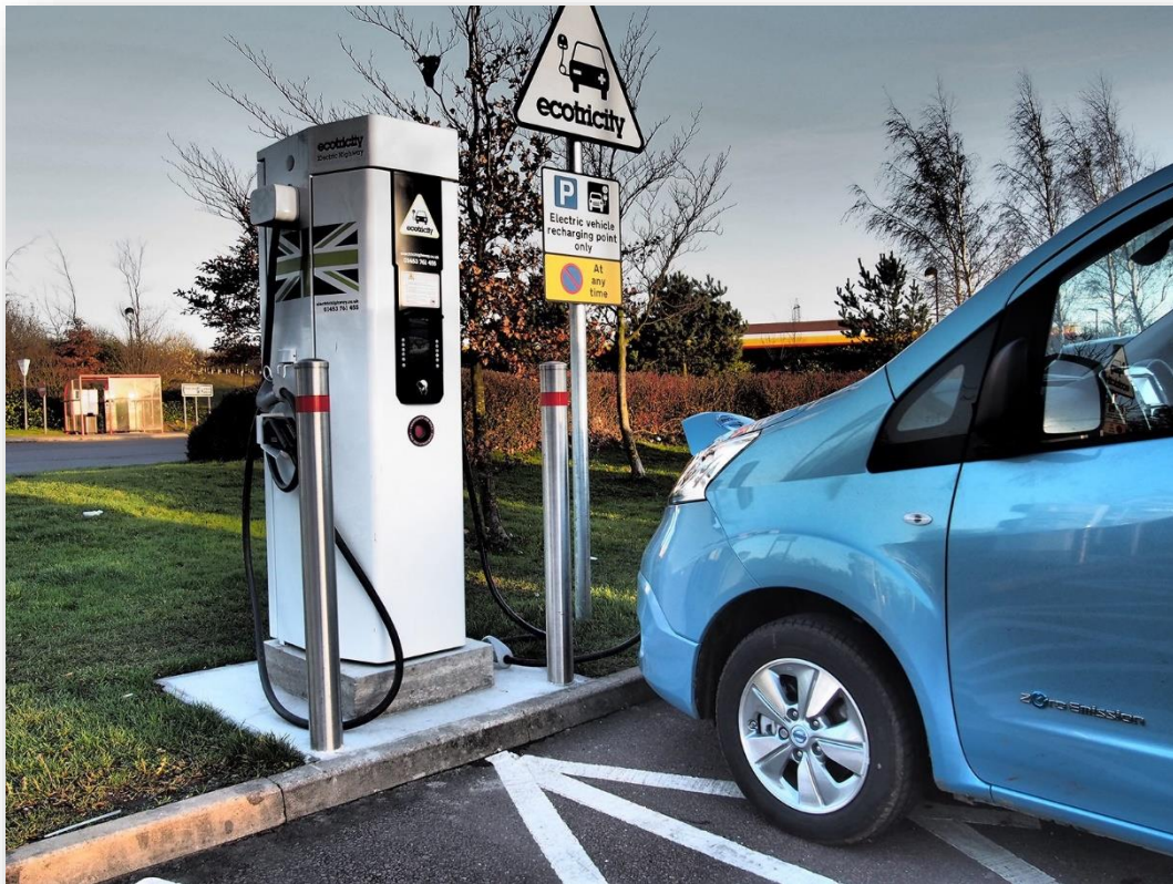
FIGURE 8: ELECTRIC VEHICLE CHARGEPOINT
