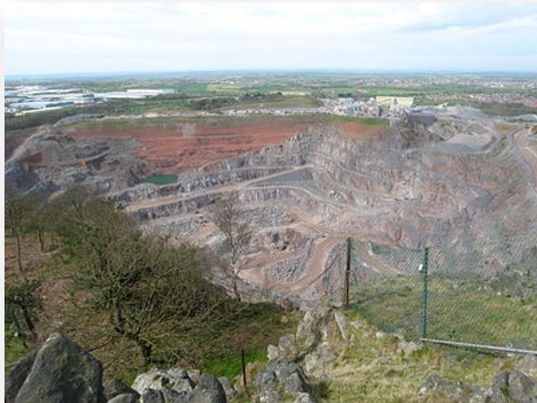
FIGURE 19: BARDON HILL QUARRY
