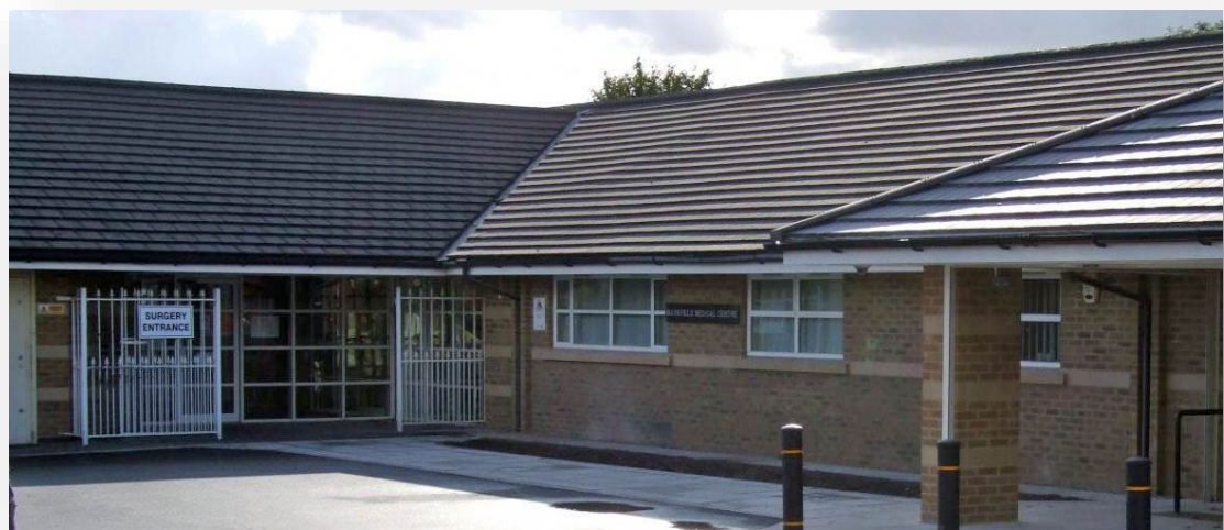
FIGURE 13: MARKFIELD MEDICAL CENTRE
