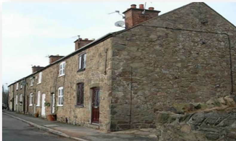
FIGURE 11: NEW ROW, HILLSIDE
