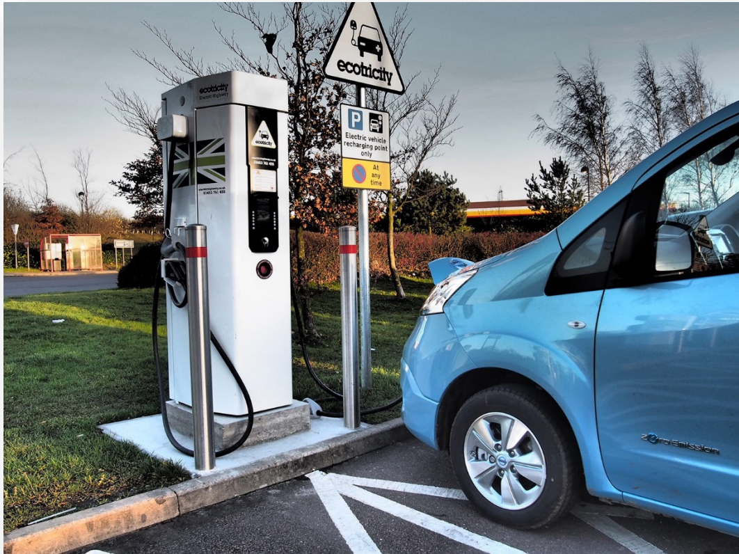
FIGURE 8: ELECTRIC VEHICLE CHARGEPOINT
