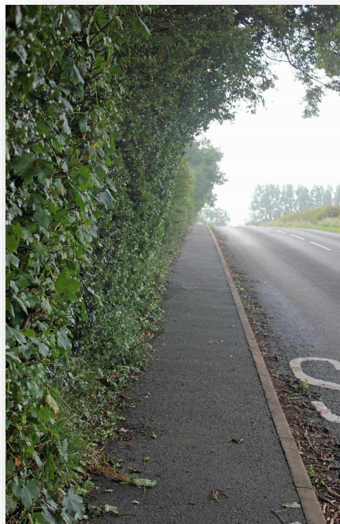
FIGURE 21: NARROW PAVEMENT ALONGSIDE LONDON ROAD
