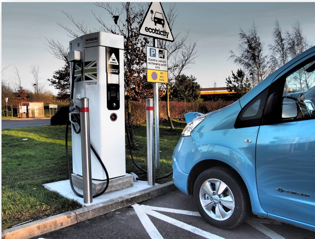
FIGURE 8: ELECTRIC VEHICLE CHARGEPOINT
