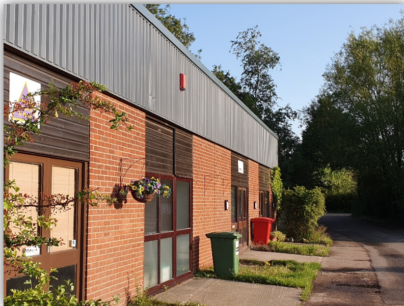
Figure 21: Willow Park Industrial Estate
