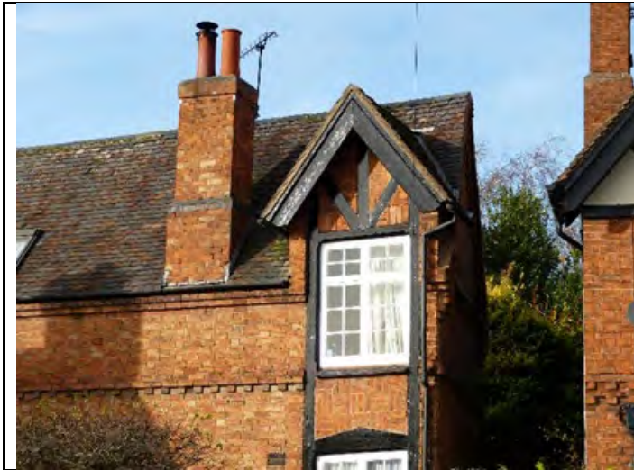
Brick infill panels within timber framing
