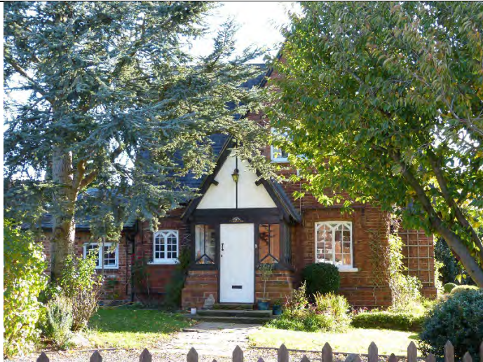
White painted gothic style timber casement windows
