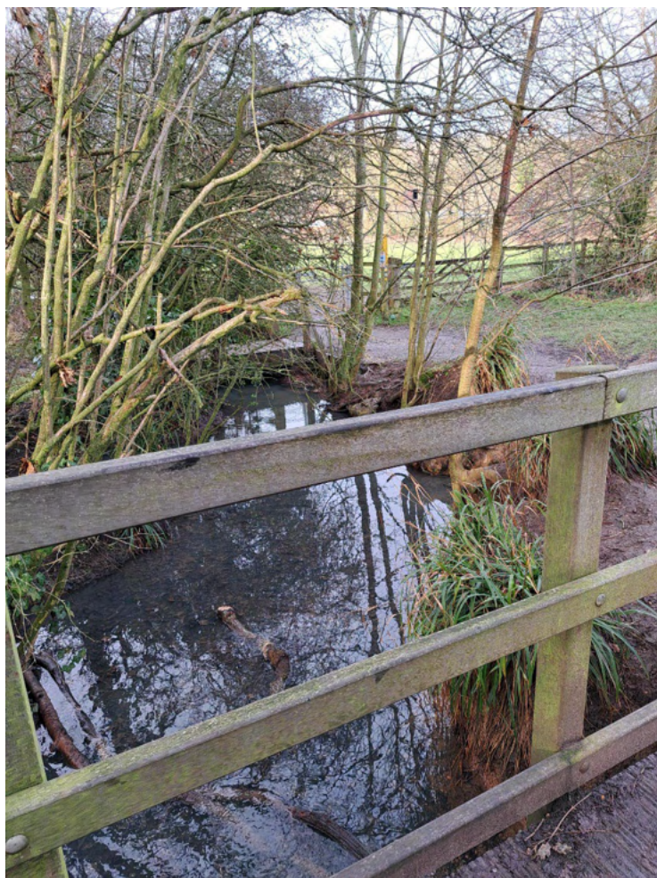
Figure 6: Watercourse through Burbage Wood
