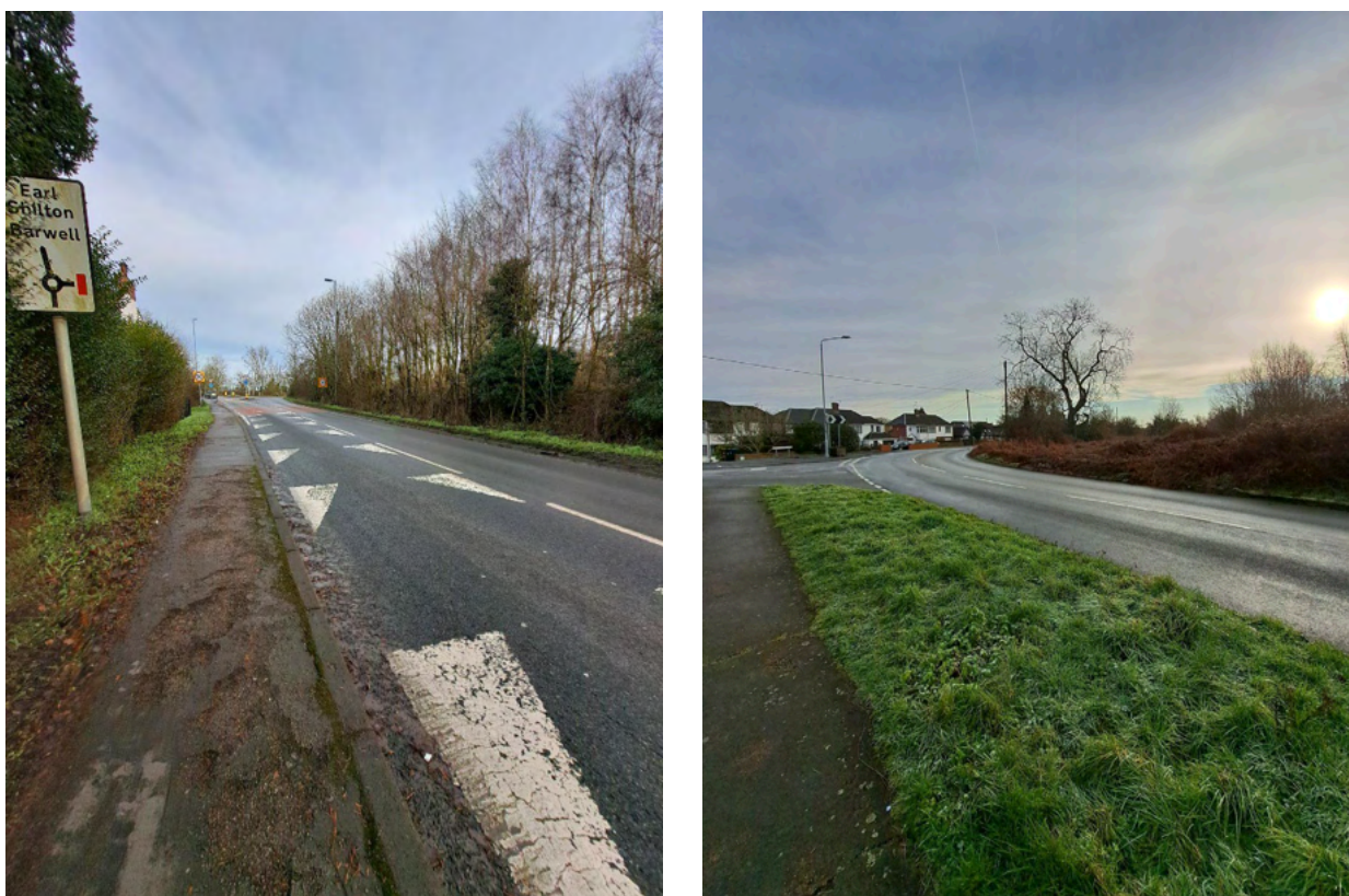
Figure 22: Images showing tree lined belt along Leicester Road edge and Elvesthorpe Lane which runs through Area D, dividing the larger and smaller portions of the area
