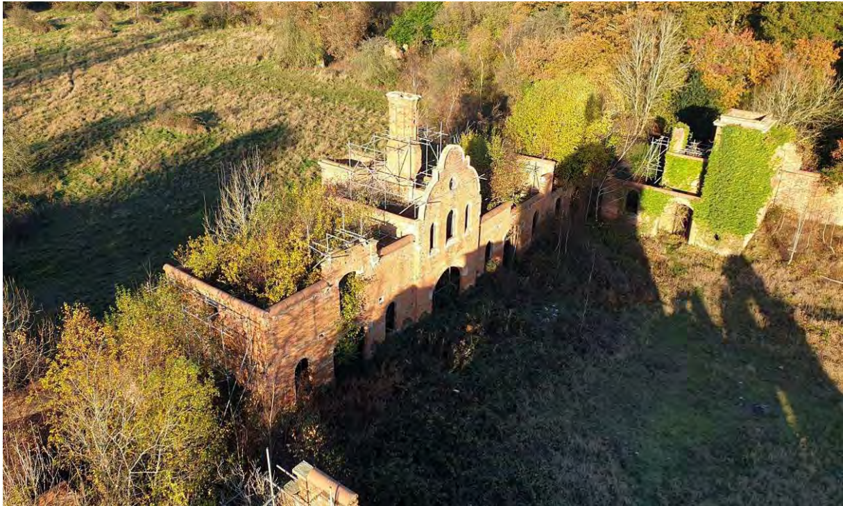
Photograph 4: West range - east facing elevation at an angle, as seen from the cherry picker
