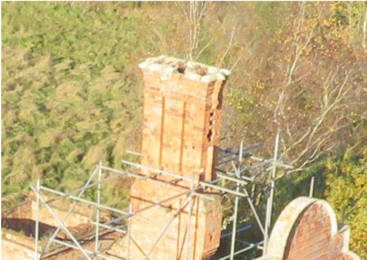
Photograph 25: Head of chimney Room 4, 4a, 4b and 4c
