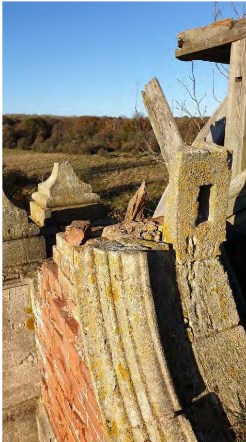
Photograph 49: Head of opening to tower to south side
