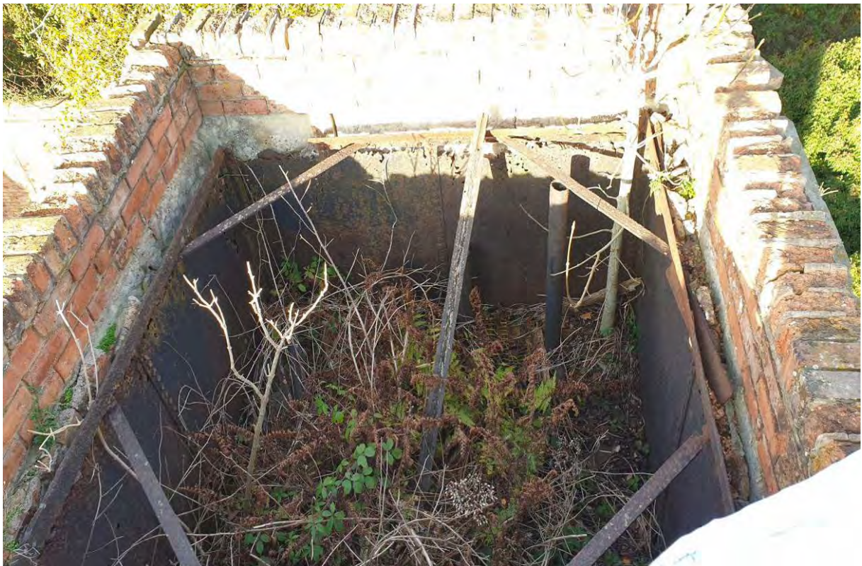
Photograph 16: Former water tank as seen from the cherry picker (north range - area '10')
