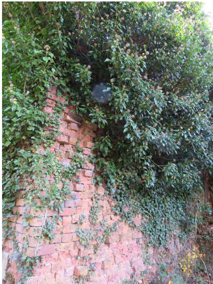
Photograph 32: West wall of Room 9a
