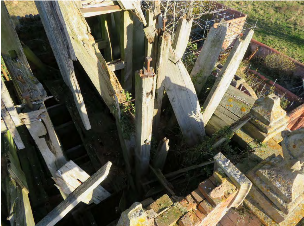
Photograph 46: Tower roof structure
