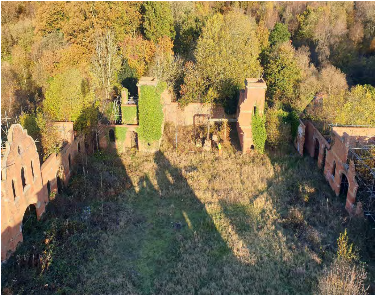
Photograph 5: North range - south facing elevation, as seen from the cherry picker
