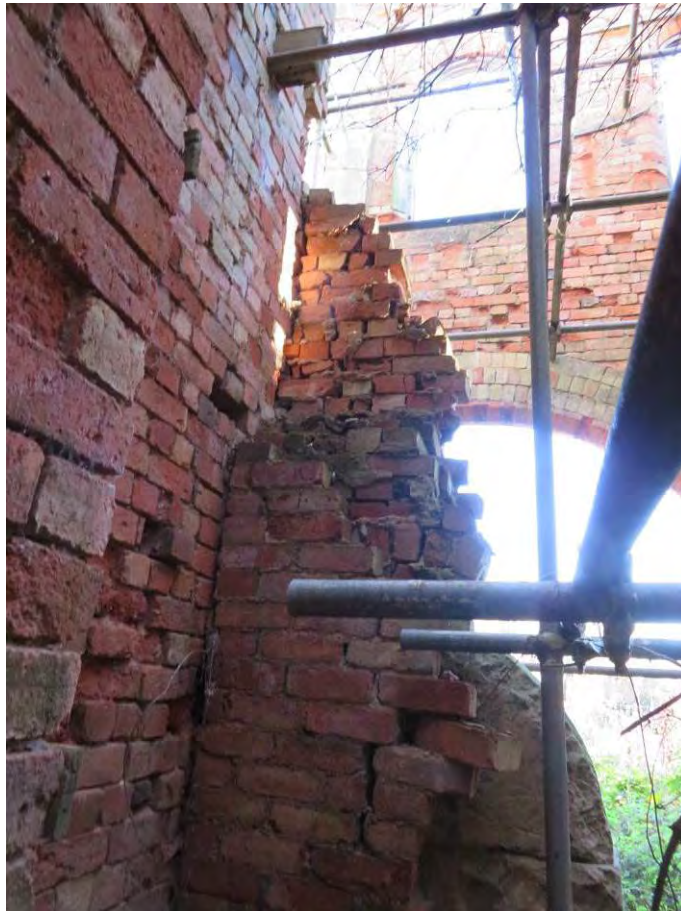
Photograph 29: Brickwork to niche to Room 4
