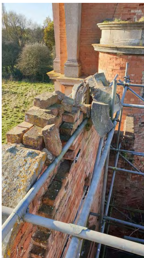
Photograph 40: Head of south gable to Room 20
