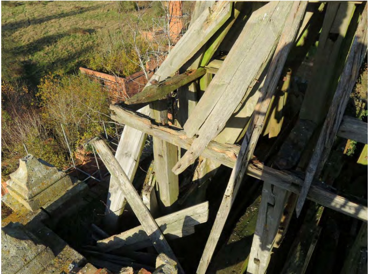
Photograph 44: Tower roof structure
