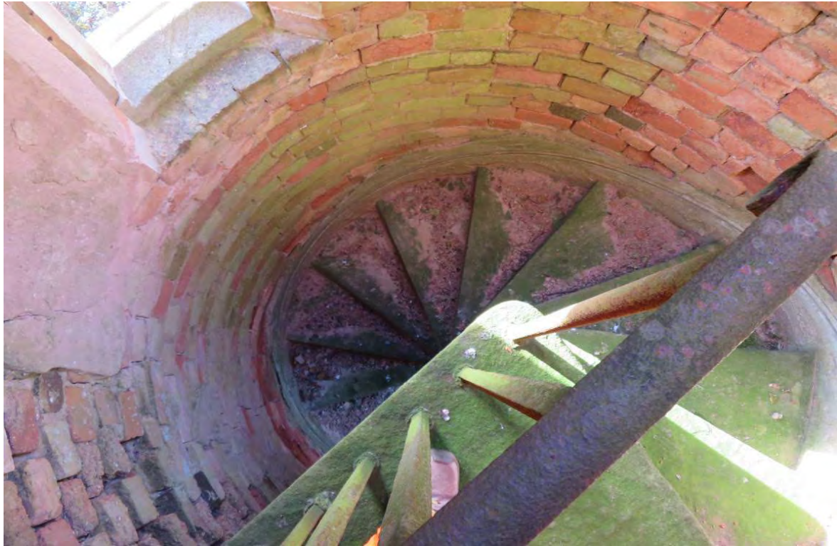
Photograph 23: Stone steps to tower stair (south range)
