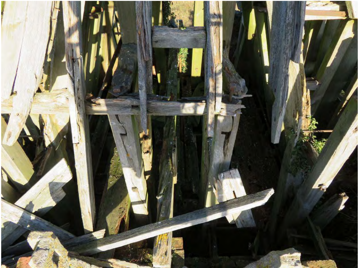
Photograph 47: Tower roof structure
