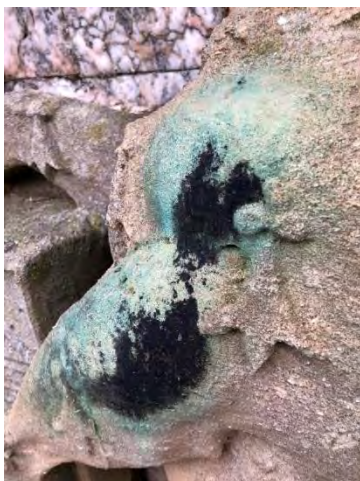
Plate 16: – detail of the sinister unicorn's proper left front leg shoulder showing a curious pattern of staining associated with the copper run-off from the horn. This is also reflected on the dexter unicorn.
