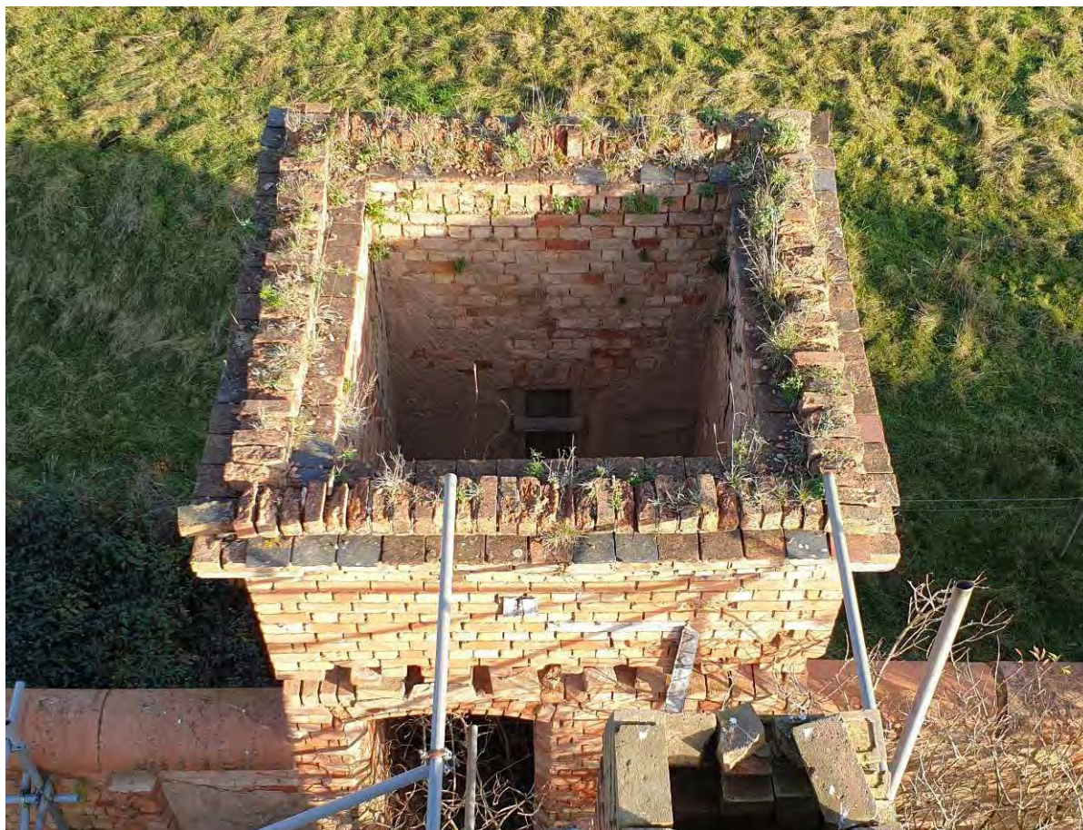
Photograph 37: Tower to Room 15b
