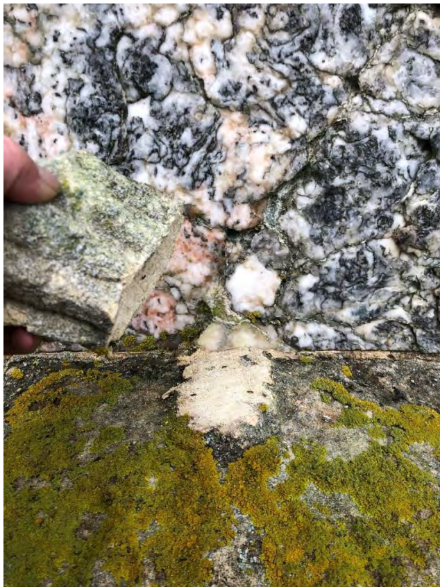
Plate 9: The upper surface of the coronet. There is a particularly heavy build-up of lichen here.
