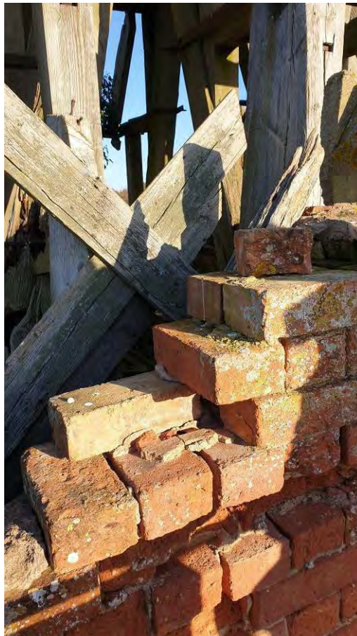
Photograph 50: Brickwork to head of tower Room 21
