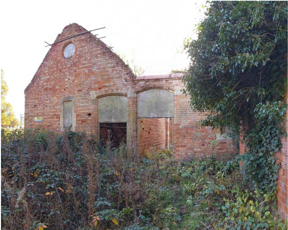
Photograph 35: North gable to Room 11
