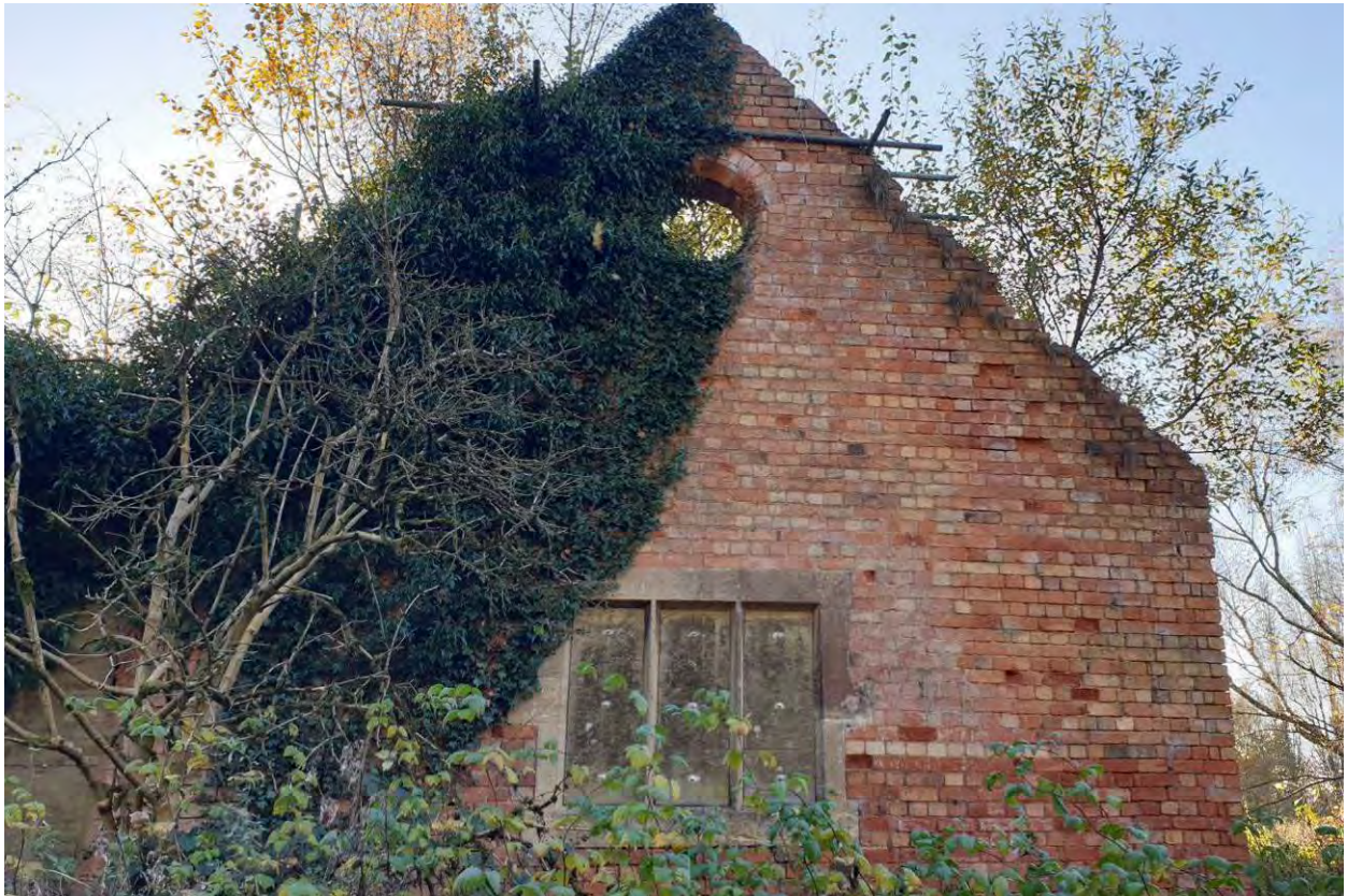
Photograph 31: North gable of Room 7
