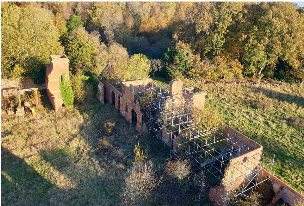
Photograph 6: East range - west facing elevation at an angle, as seen from the cherry picker
