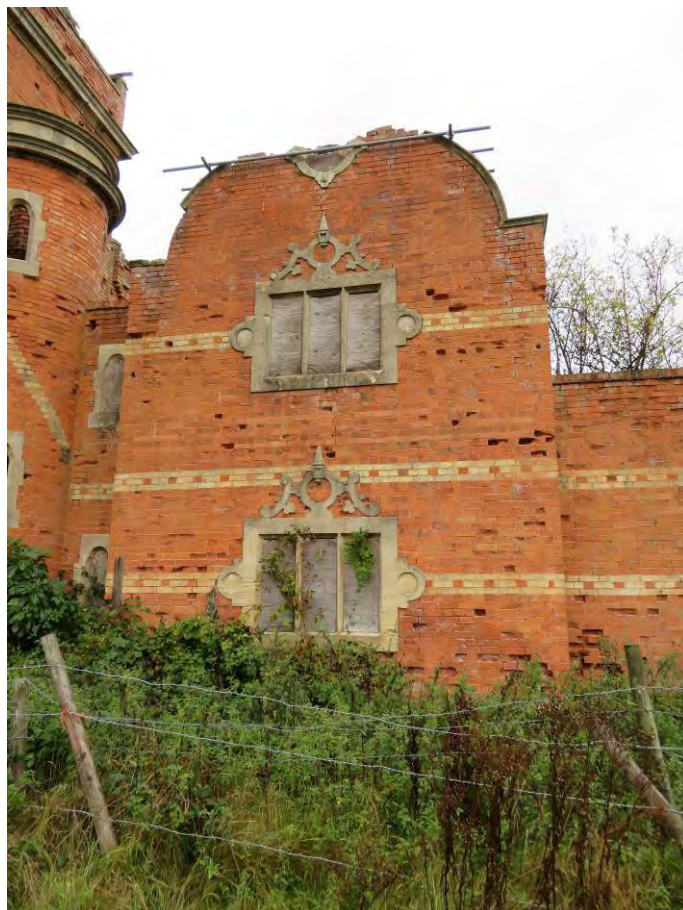
Photograph 39: South gable to Room 20
