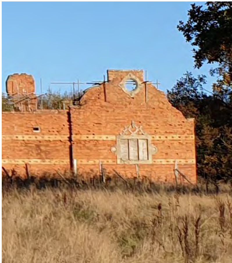
Photograph 38: South gable to Room 18
