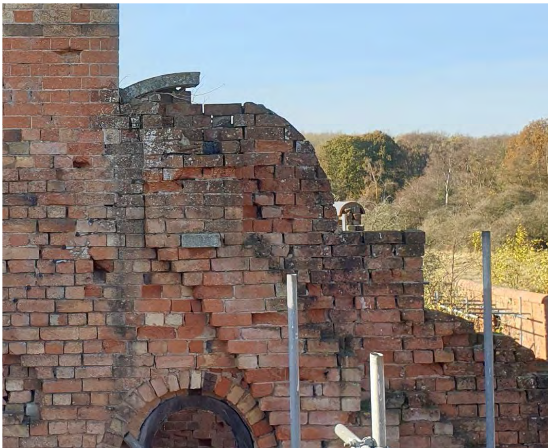
Photograph 53: Head of gable to Room 20 to west side
