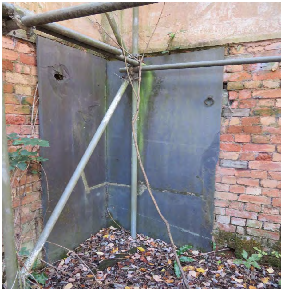
Photograph 20: Surviving slate backing for stables
