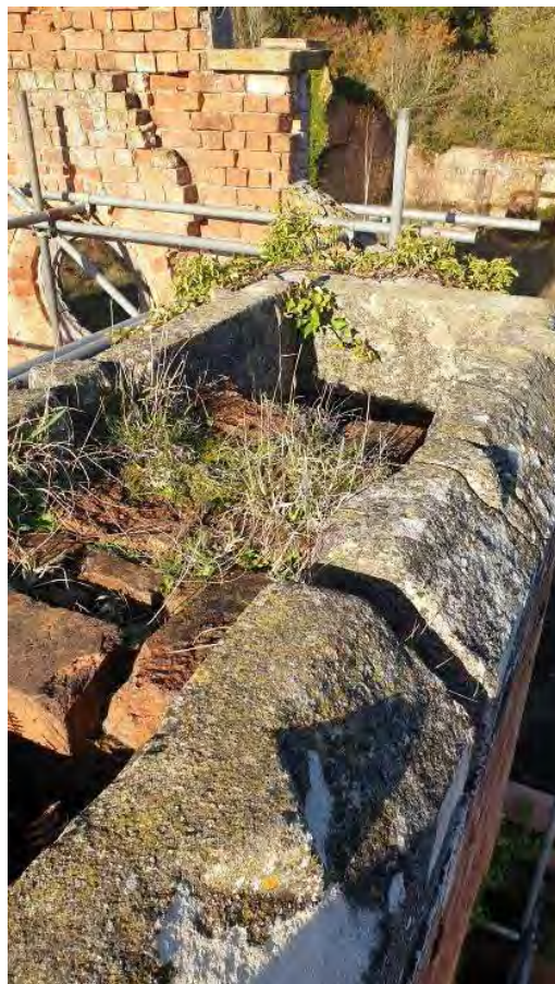
Photograph 42: Chimney to east side of Rooms 20a and 20b
