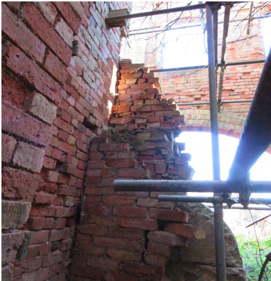
Photograph 24: Brickwork behind niche found to be loose in area '4' (refer to TMP diagrammatic plan)
