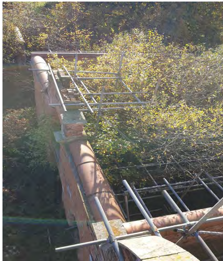
Photograph 14: Coping tiles from previous works to mitigate water ingress into the masonry fabric (west range - east elevation)
