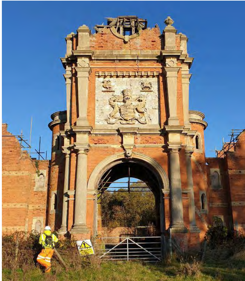
Photograph 2: South range tower - south facing elevation
