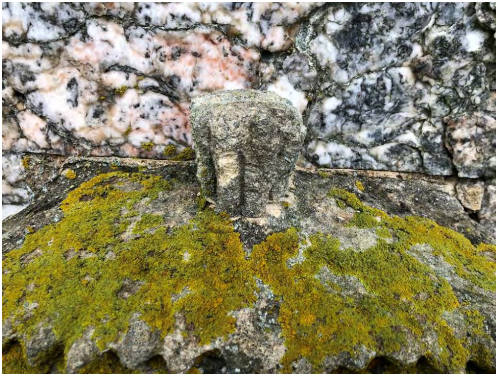
Plate 9: The upper surface of the coronet. There is a particularly heavy build-up of lichen here.
