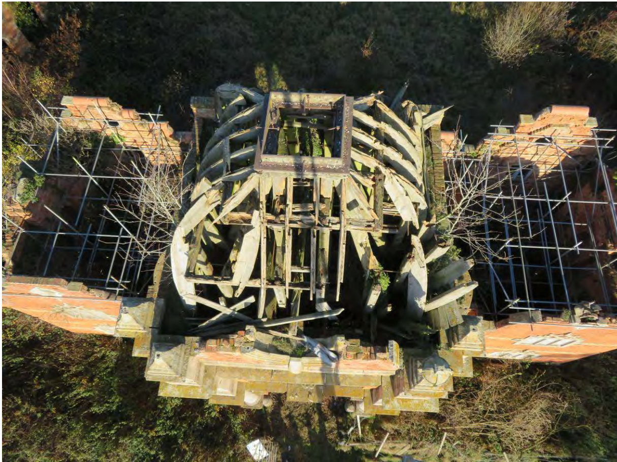
Photograph 3: South range tower - remaining timber roof, as seen from the cherry picker
