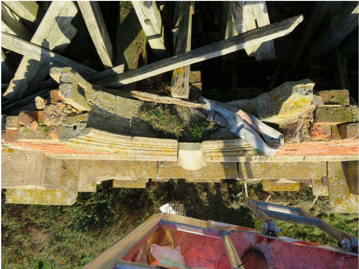
Photograph 45: Tower roof structure
