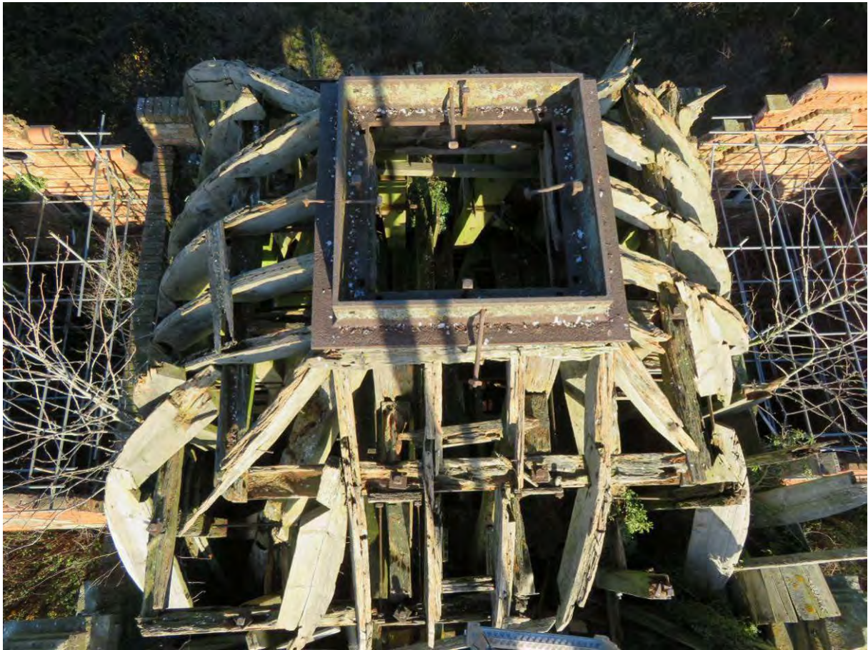
Photograph 43: Tower roof structure
