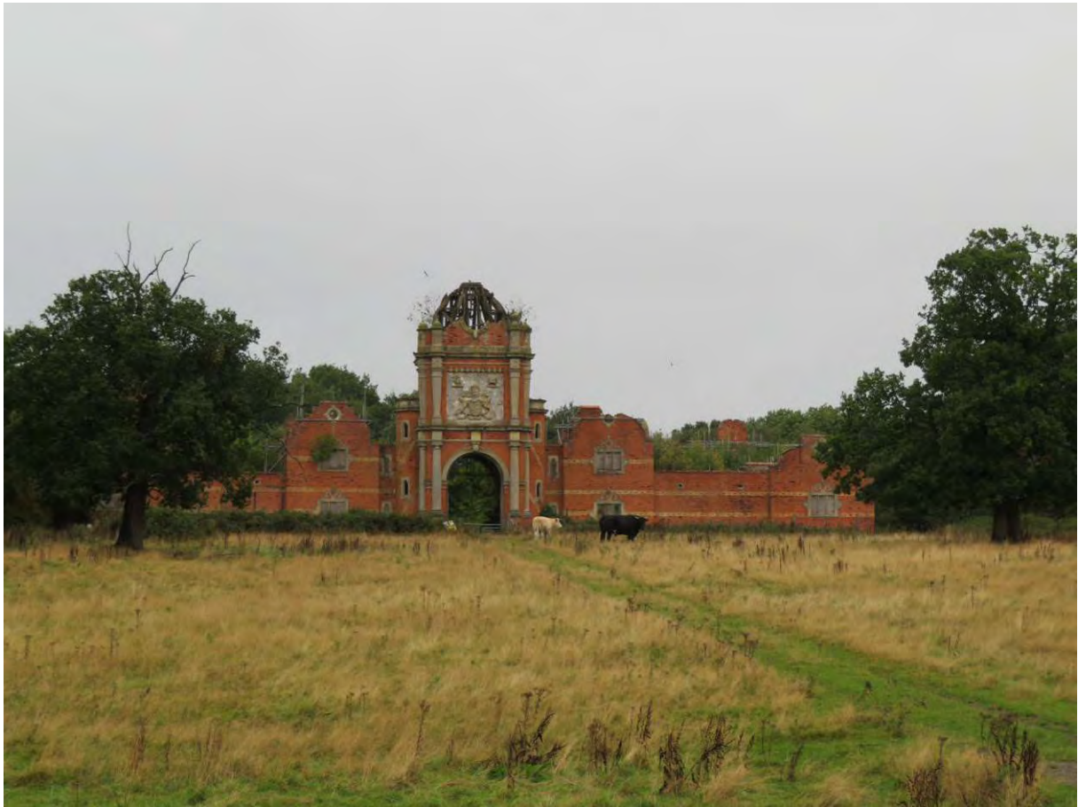
Photograph 1: South range - south facing elevation
