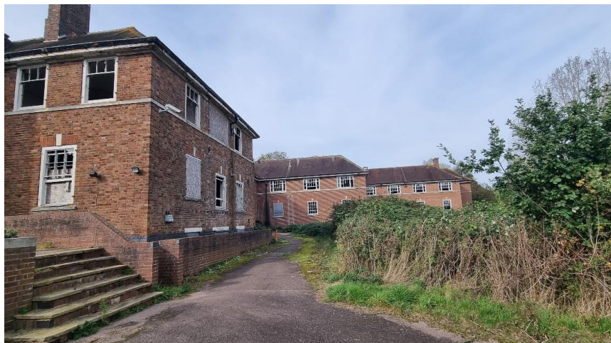
Figure 43: Photograph of extension to Bradgate House built for offices.
