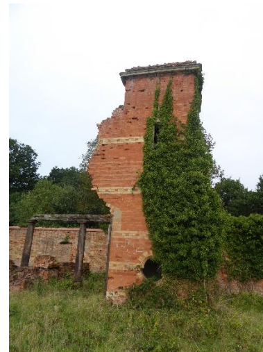
View from south of former carriage house
