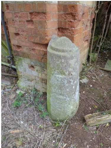
Jostle stone in main entrance
