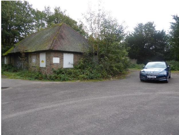
Garage and tarmac area
