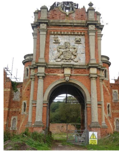
South façade, central entrance
