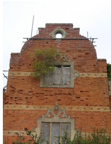
Dutch gable in south range, internal elevation
